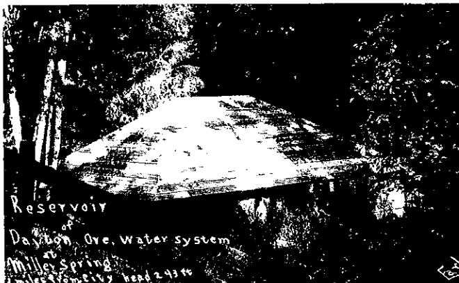
Reservoir of Dayton water system at Miller Spring three miles from city, head 243 feet, no date given. [BB]
