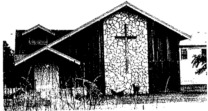
Remodeled Unionvale Church 1980 [Q].
