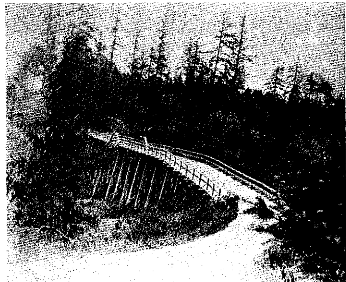
Bridge over Palmer Creek, Webfoot Road [L]
