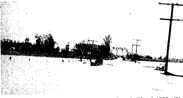
Taken from bridge looking toward railroad. Flood 1923. [I].
