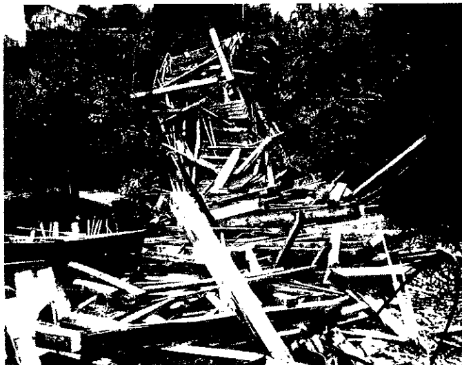
Collapsed bridge over Yamhill River at Dayton, view looks across river toward town, with "White Warehouse" at left. 1910-1915? [C].
