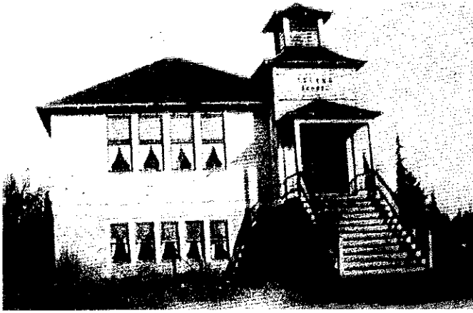
Grand Island School District #94 around 1912. Used until 1952. [FF].
